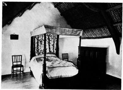
Kennixton: a bedroom. Note the plaited wheat-straw mats which form the underthatch of the roof. These are a feature of the house.
